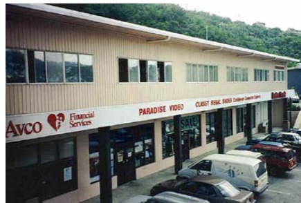
Automobile oriented buildings with little architectural detailing and extensive flat roofs are prohibited.
